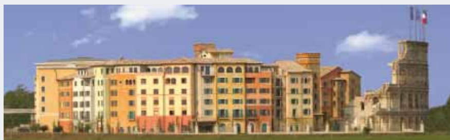
The general planning firm CHP used Allplan to design an Italian town in the Europapark Rust.
